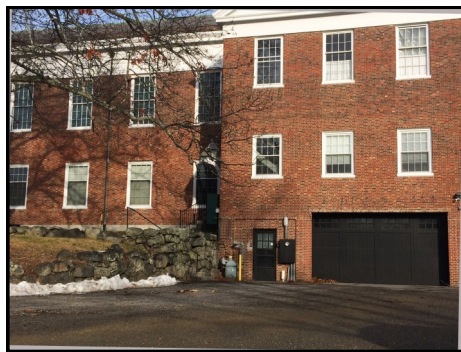
The current Town Hall side view shows garage bays and office door.
