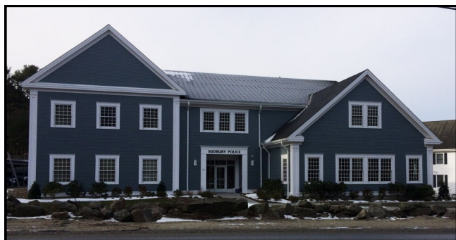
The new grey and white Police Headquarters is next to the white Fire Department Headquarters.
